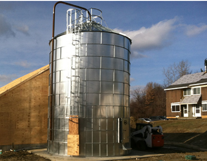
Above: Wood pellet boiler at Montpelier Senior Housing; Wood pellet silo at Applegate, Bennington
